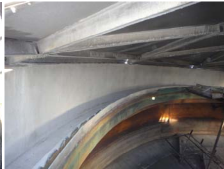
Existing Sludge Thickener- After Surface Preparation and Concrete Rehabilitation
