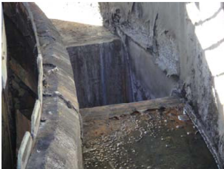
Existing Sludge Thickener
