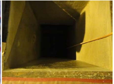
Existing Influent Channel After Coating Application
