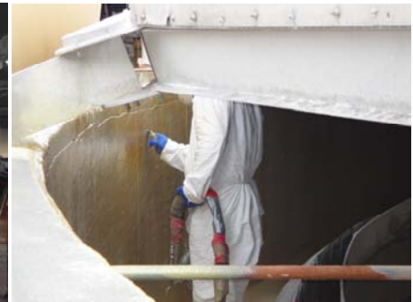
Existing Sludge Thickener During Coating Application
