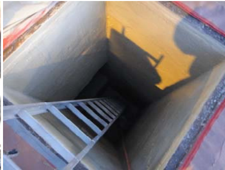
Existing Influent Channel - After Surface Preparation and Concrete Rehabilitation
